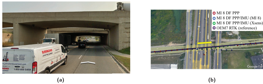
FIGURE 10 Photograph and aerial view of trajectory for Underpass B: (a) is a Google Earth view of the underpass and (b) is a Google Earth view of the trajectories for the three sensor fusion strategies.
